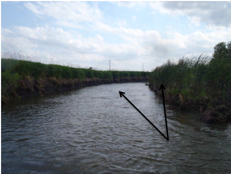
Figure 37. Bank erosion near 11MS022
