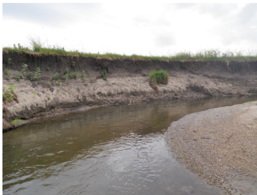
Figure 33: Severe bank erosion at sites 11MS016 (Left) and 11MS121 (Right) along Chanarambie Creek (10170204-522)
