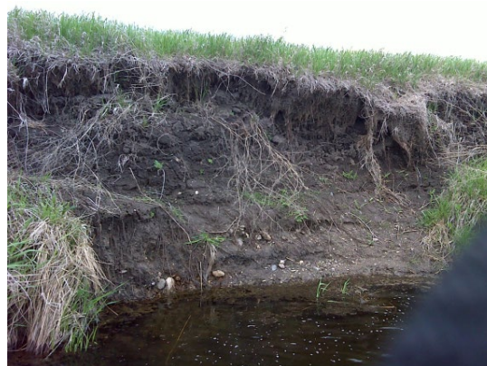
Figure 34: Eroding bank at site 11MS123 along North Branch Chanarambie Creek (10170204-560)
