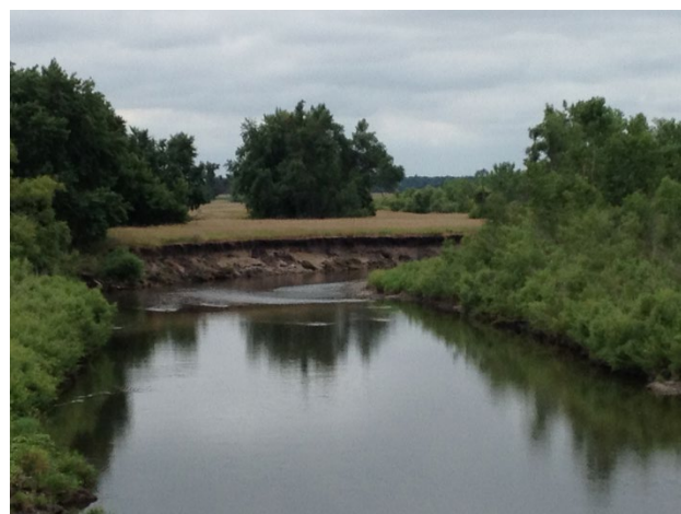
Figure 93: Eroded bank at 11MS001 along Rock River (10170204-501)
