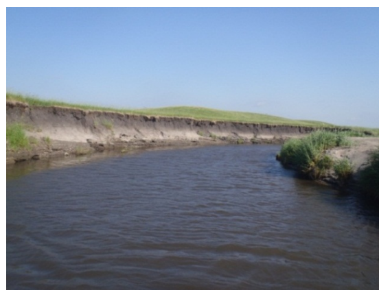
Figure 81: Heavy bank erosion at 11MS002 along Little Rock River (10170204-513)
