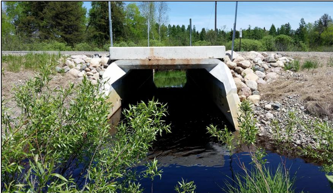
Photo 1. The new culvert on Wouri Road.
