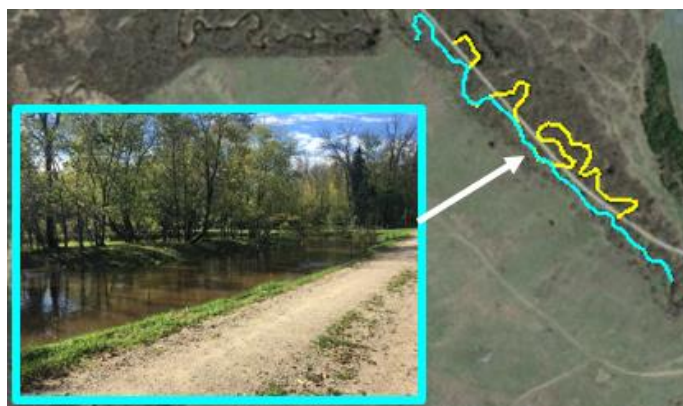
Figure 12. Channelized section (blue line) of the Blackduck River that occurred prior to 1939, reducing the historical stream (yellow line) length by 34% and increasing stream slope by 60%. The photo shows the channelized reach along the roadway.
