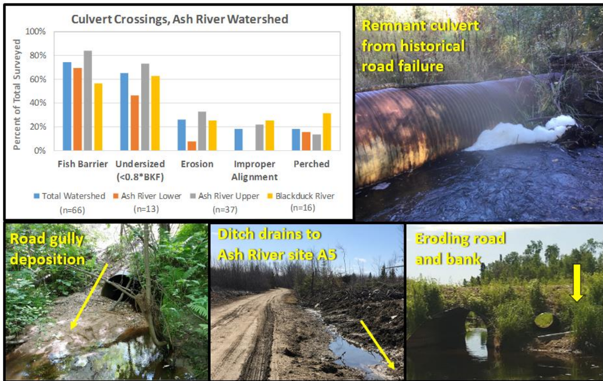
Figure 13. Culvert inventory results (Top Left) in the Ash River Watershed identifying the most commonly found problems at stream-road crossings. Photos: Examples of culverts and roadways that have contributed sediment to stream channels in the Ash River Watershed.
