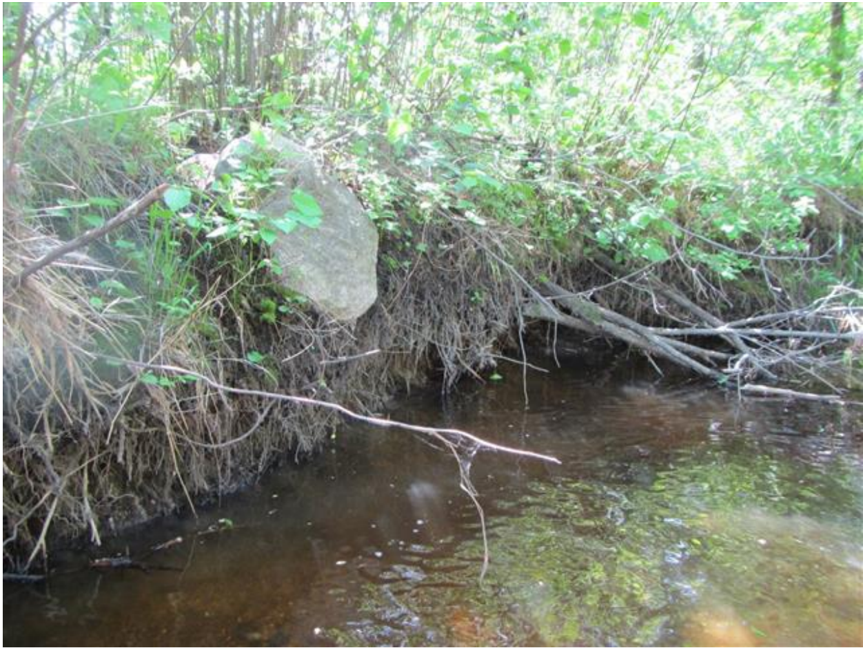
Figure 44: Picture from biological station 14RD246, taken on June 10, 2015, showing bank erosion on the Hill River.
