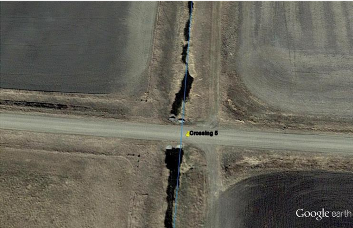
Figure 21: Crossing 5: potential fish barrier, especially under low flow conditions. In this photo, there appears to be no water flowing through the culverts. Imagery taken on 4/14/2015.
