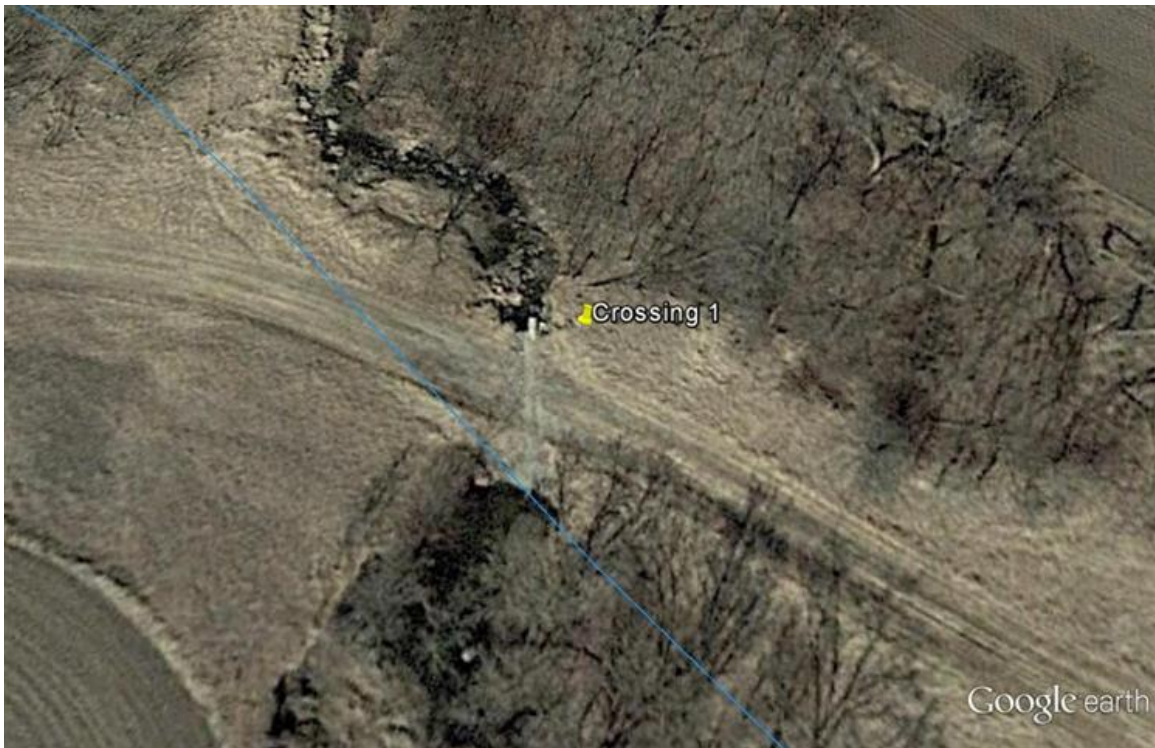
Figure 17: Crossing 1: potential fish barrier (if white pipe in photo is the only flow path under the road). Imagery taken on 4/14/2015.
