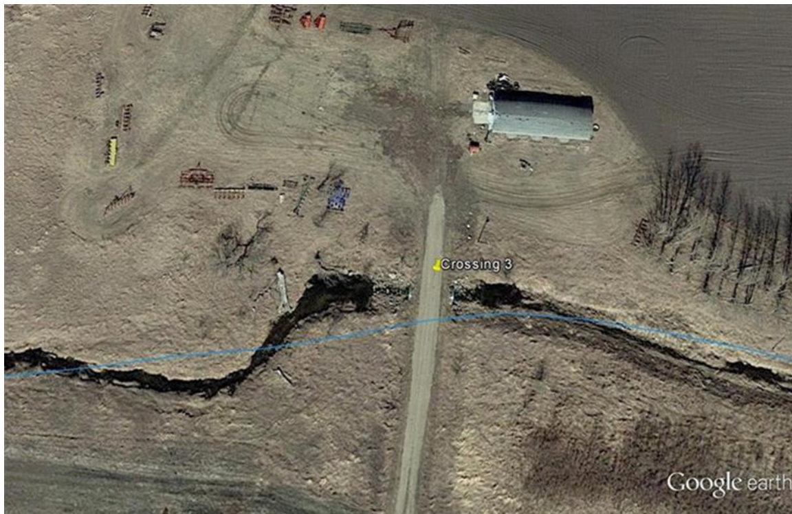
Figure 19: Crossing 3: potential fish barrier, especially under low flow conditions. Imagery taken on 4/14/2015.
