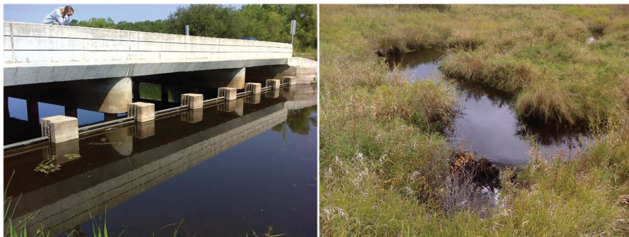
Figure 6. Images of potential connectivity barriers along AUID 646, including the Lower Rice Lake Dam at the Dam Drive crossing on July 20, 2017 (left); and a beaver dam upstream of the CSAH 36 crossing on September 28, 2016 (right).
