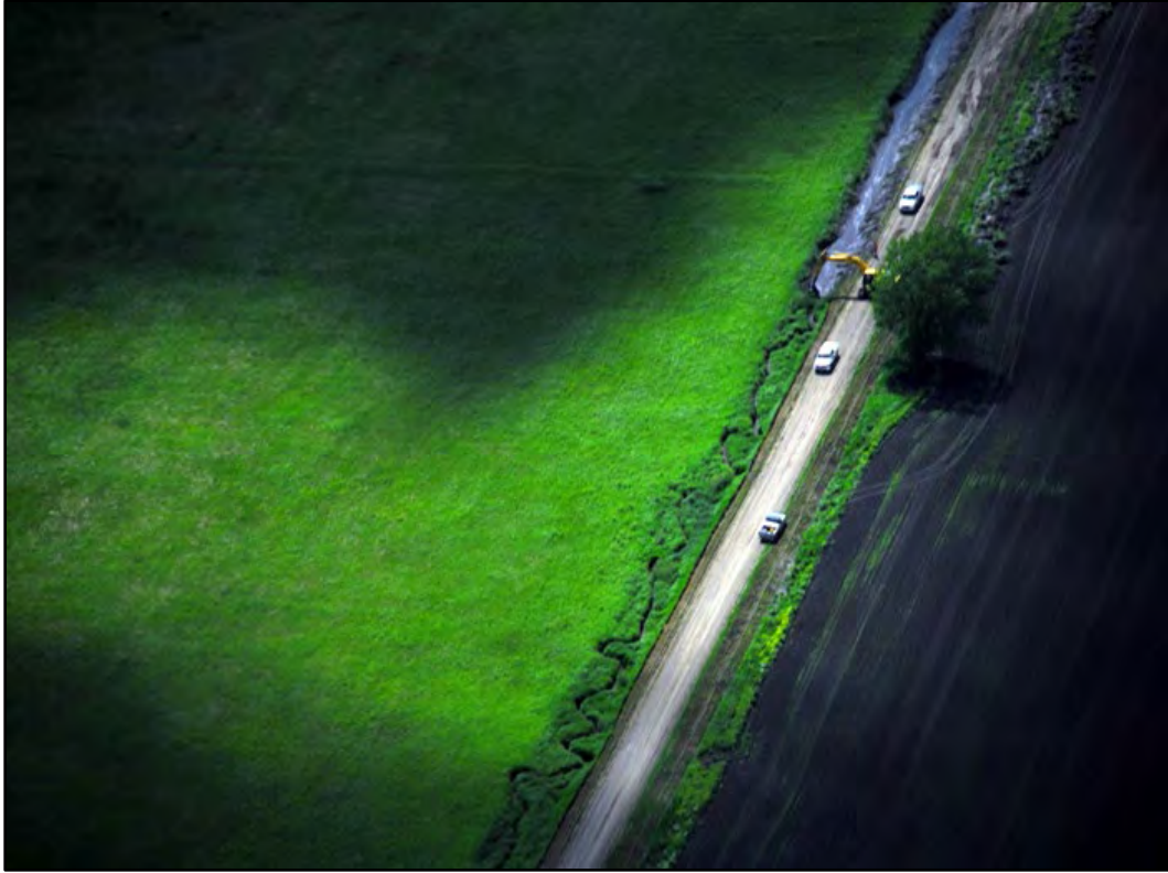
Figure 54. Ditch repair in progress.
