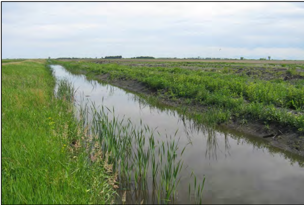
Figure 55. Photo after repair showing high width depth ratio, fine sediment, and cattail colonization.
