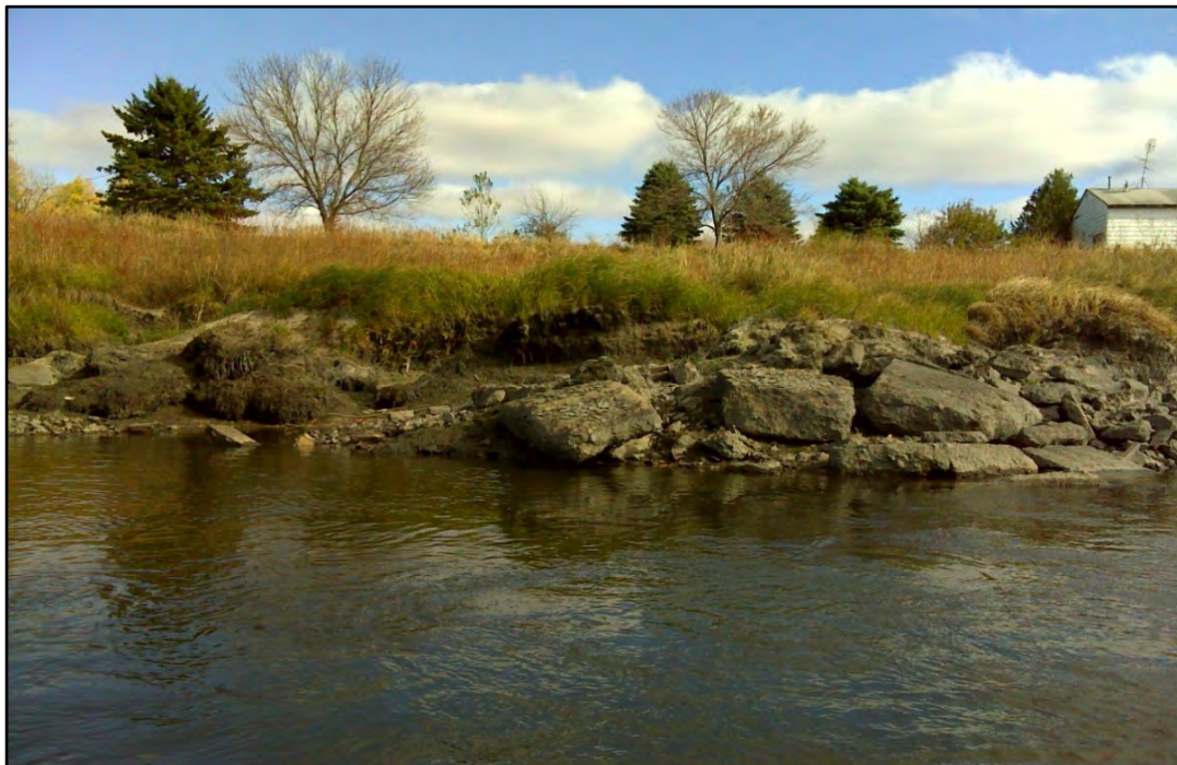
Figure 30. Failed erosion prevention efforts near waypoint 598.
