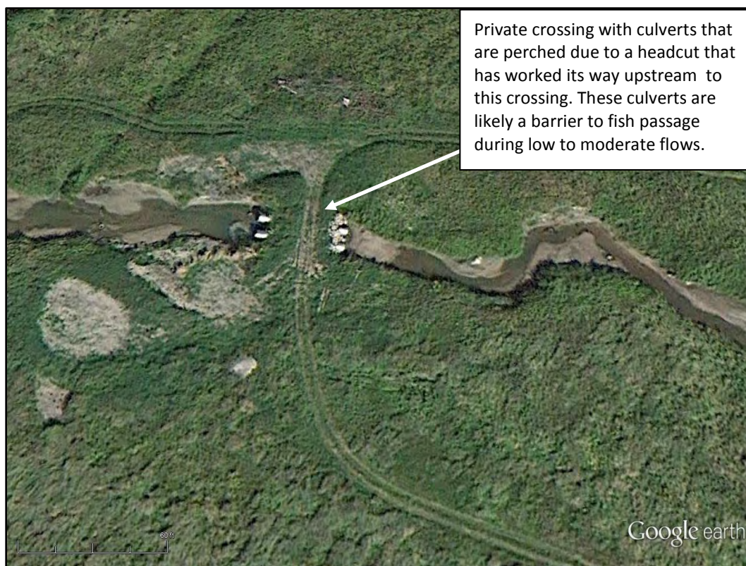
Figure 80. Google Earth photo 9/5/11 showing a pair of culverts on a private stream crossing located about 4 miles NW of Callaway that appear to be perched creating a fish passage barrier.
