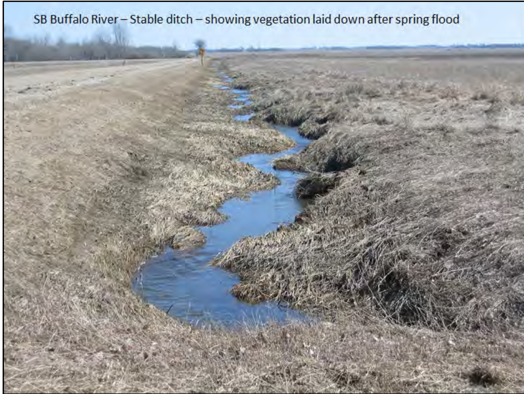
Figure 52. Low flow channel at near bank full. The meander pattern adds storage and reduces velocities.
