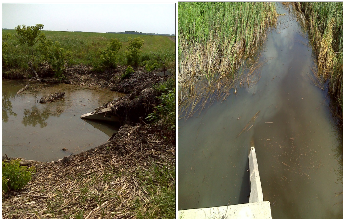
Figure 21. Upstream and downstream photos of the 250th Street crossing of CD 23.
