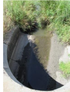
Figure 61. Low flow through culvert at S009-052.
