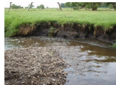
Figure 44. Bank erosion at site 14DM071.
