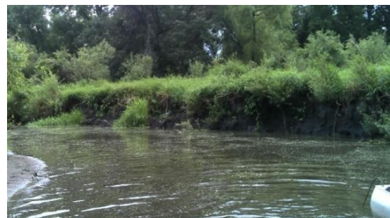
Figure 229. Bank erosion at site 14DM002.
