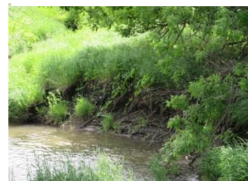
Figure 59. Bank erosion at site 14DM057.
