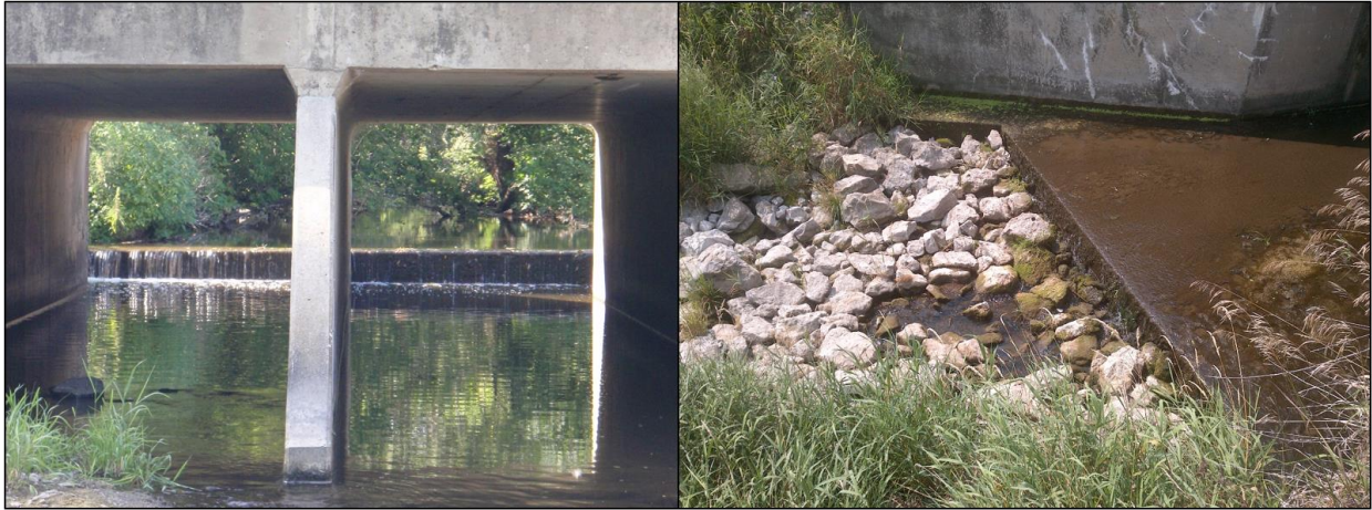
Figure 5: Fish migration barriers at stations 09CD072 (left) and 09CD084 (right).
