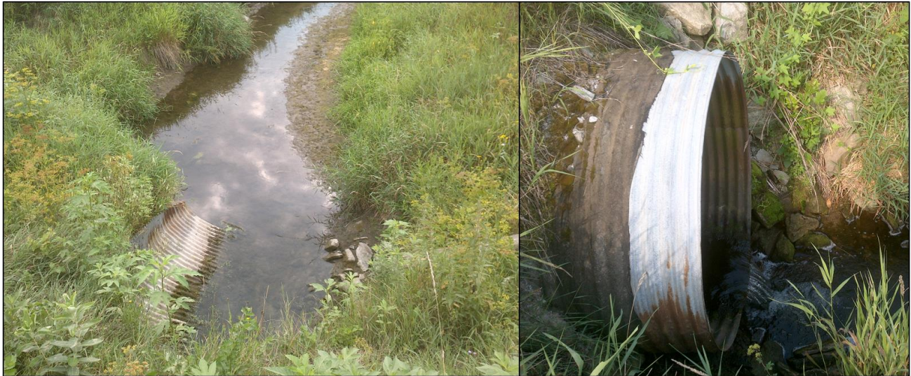
Figure 6: Low flow conditions (left) and a perched culvert (right) documented in 2021 on County Ditch 65; both have the potential to negatively impact fish migration. The perched culvert is located just upstream of AUID -529 at the 255 th Street crossing.
