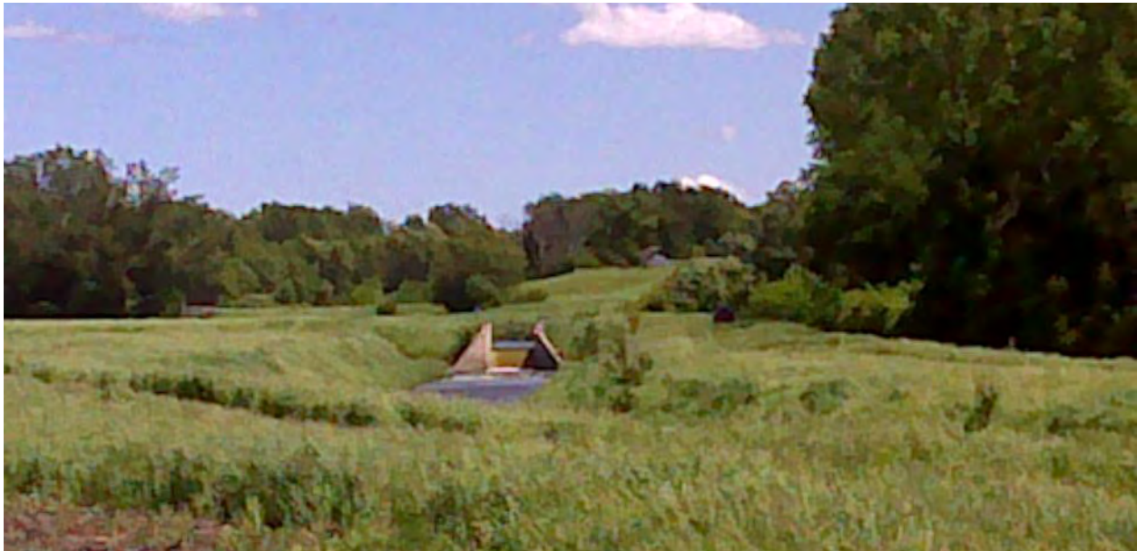
Figure 47. View of structure on County Ditch 6 from Twp Hwy 111 looking upstream
