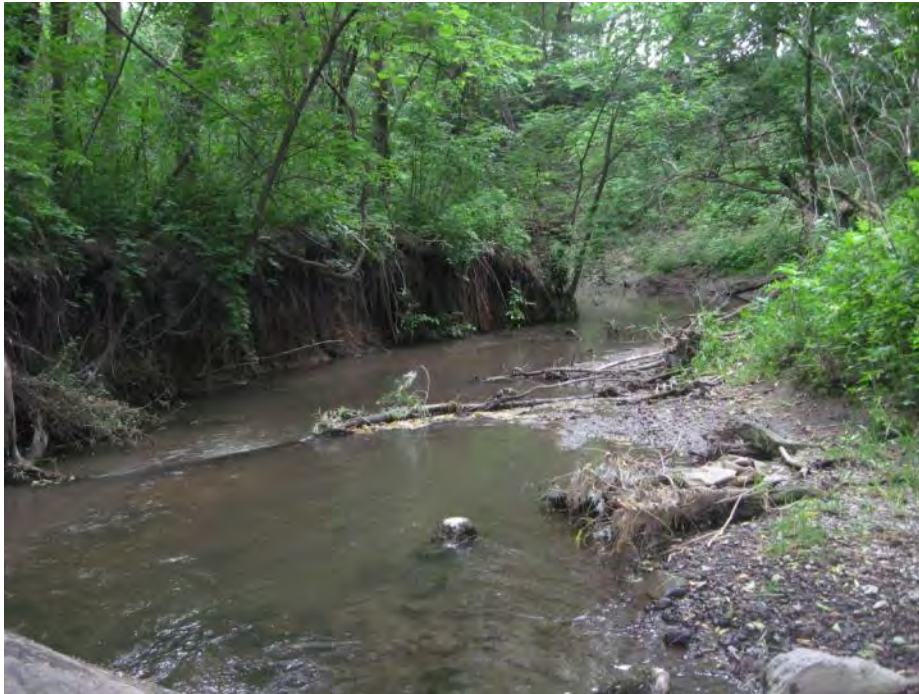
Figure 39. Photograph of station 08MN020 showing eroding banks.
