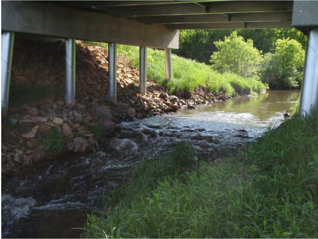
Figure 36. Riffle under bridge near biological station 08MN027
