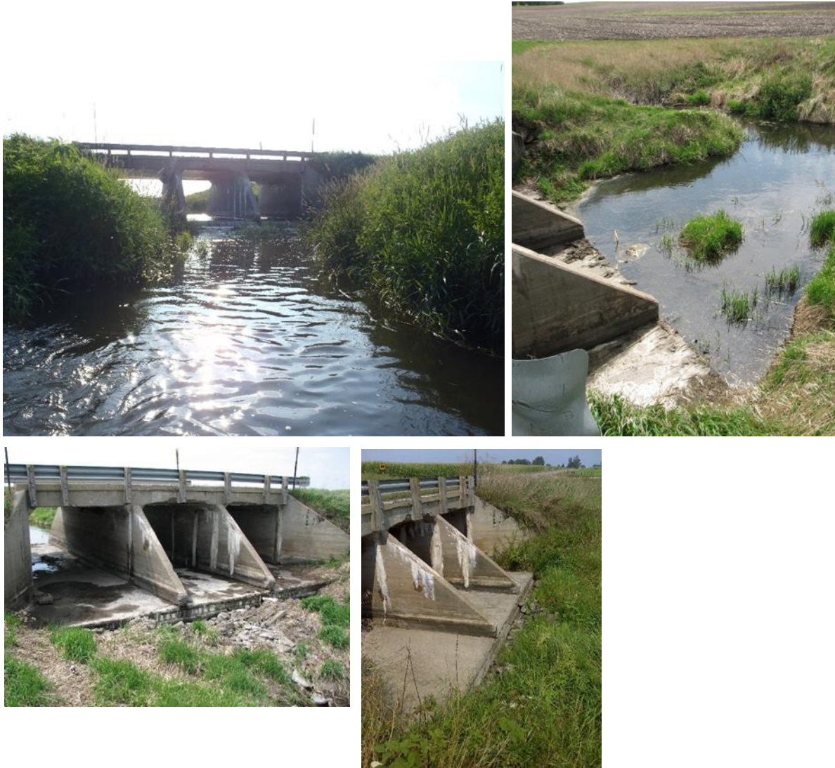
Figure 250. Biological station 13MN139 (July 10, 2013) fish barrier (upper left); (May 1, 2015) intermittent flow fish barrier (upper right and lower left); (September 1, 2015) no flow (lower right).
