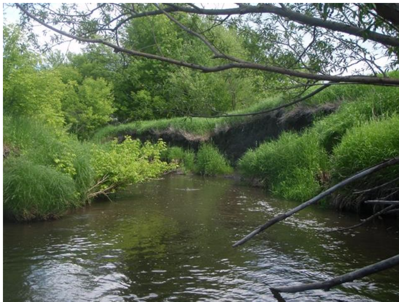
Figure 77. Biological station 13MN165 (June 11, 2013) stream bank erosion.
