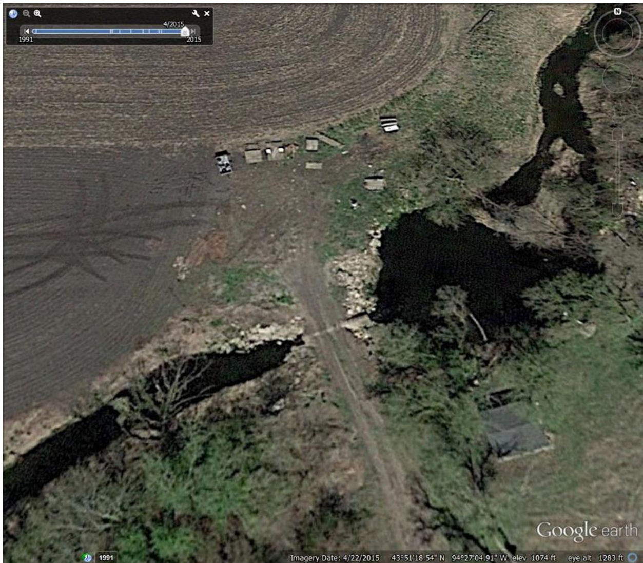
Figure 217. Google Earth aerial image of Mink Creek 'homemade' stream crossing. Culvert appears undersized causing downstream scouring.
