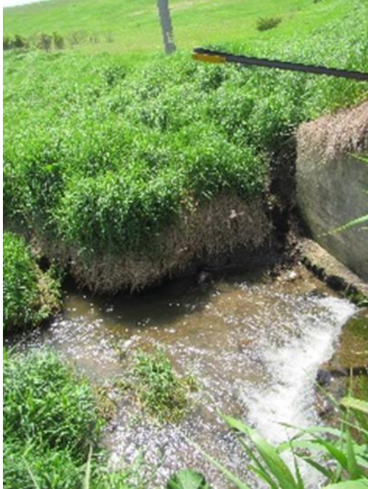
Figure 28. Biological station 91MN08 (May 24, 2016) barrier downstream side of culvert.
