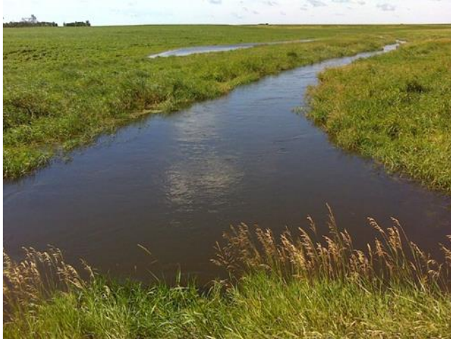
Figure 247. Spring Branch Creek at 360th St. (July 14, 2016) stream field connection.
