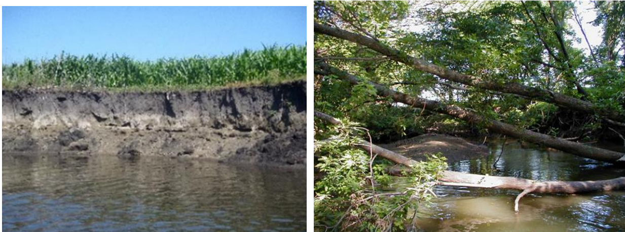
Figure 203. Biological station 13MN142 (July 17, 2013) eroded stream bank with narrow buffer (left); biological station 90MN099 (August 1, 2008) incised channel and sediment deposition (right).
