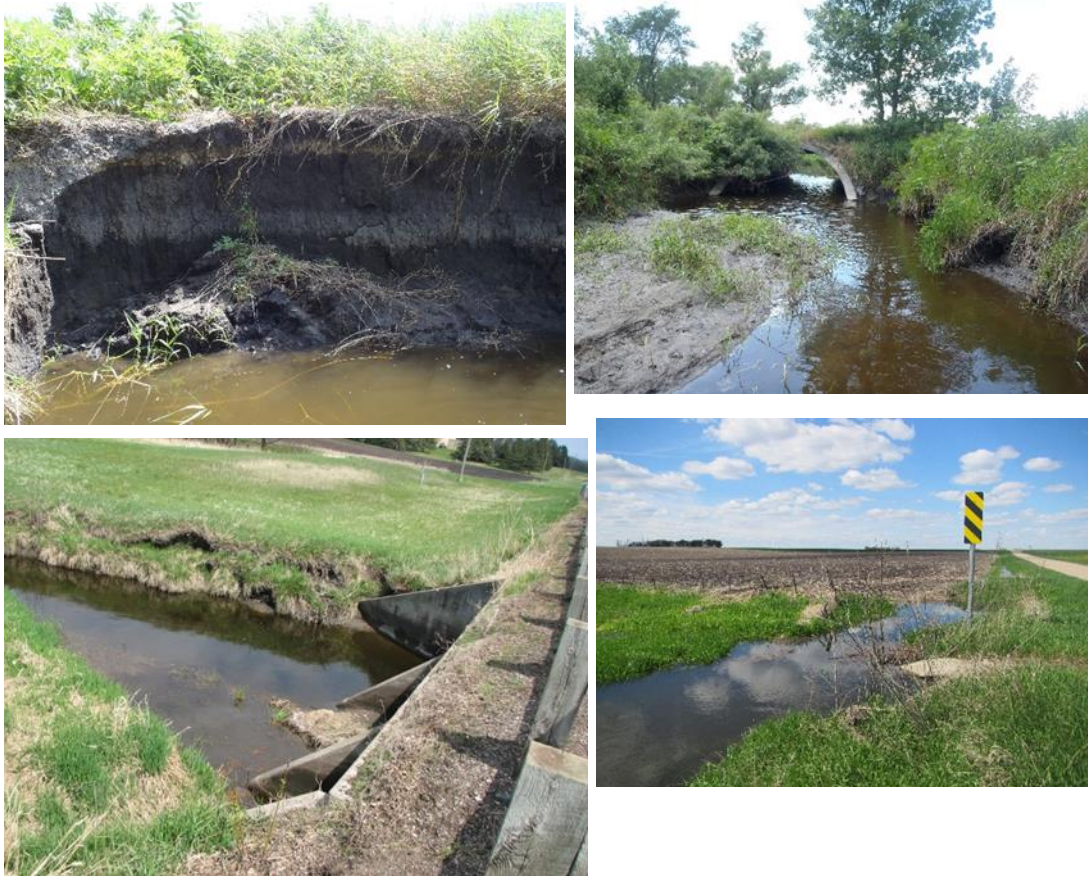
Figure 230. Biological station 13MN143 (July 22, 2014) stream bank erosion (upper left); sediment deposition (upper right); bank sloughing (lower left); (May 2, 2016) stream field connection (lower right).
