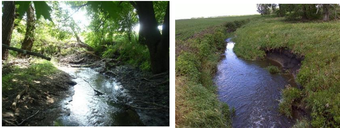
Figure 222. Biological station 13MN144 (July 10, 2013) raw banks (left); (June 2016) stream bank erosion (right).
