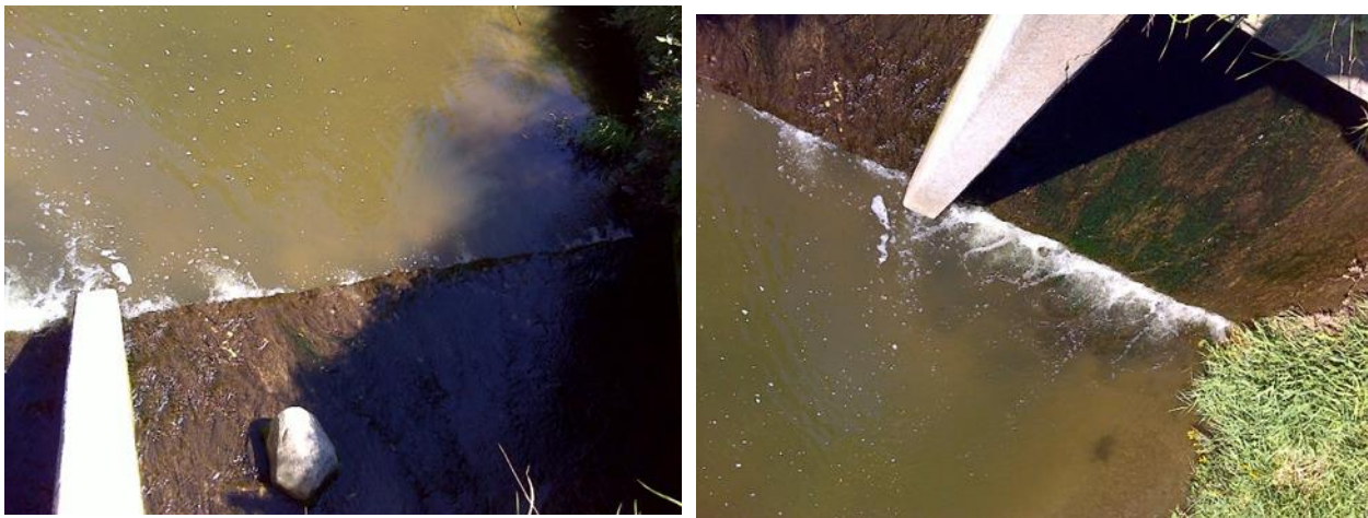
Figure 120. Butterfield Creek at 640th St. (August 31, 2016) filamentous algae and perched culvert (left and right).
