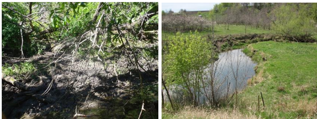
Figure 129. Biological station 13MN124 (May 1, 2015) stream bank erosion (left and right).
