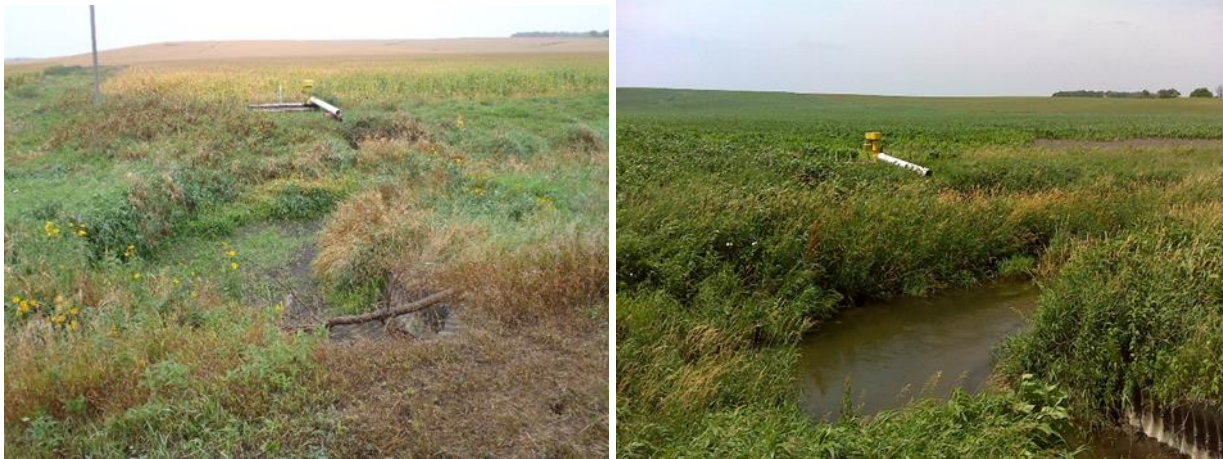
Figure 140. Biological station 13MN154 (September 12, 2012) dry streambed with drain tile pump (left); (July 10, 2014) water damaged field, limited riparian buffer (right).
