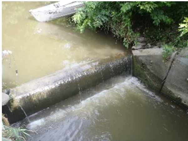
Figure 157. Biological station 13MN110 (July 23, 2013) low head dam, fish barrier.
