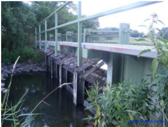
Figure 297. Lake Hanska - Dam at Outlet.
