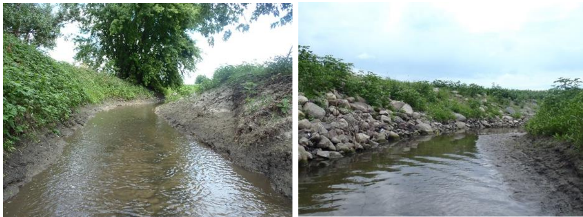
Figure 166. Biological station 13MN164 (July 23, 2013) stream bank erosion, recently cleaned out channel (left); riprap bank stabilization (right).
