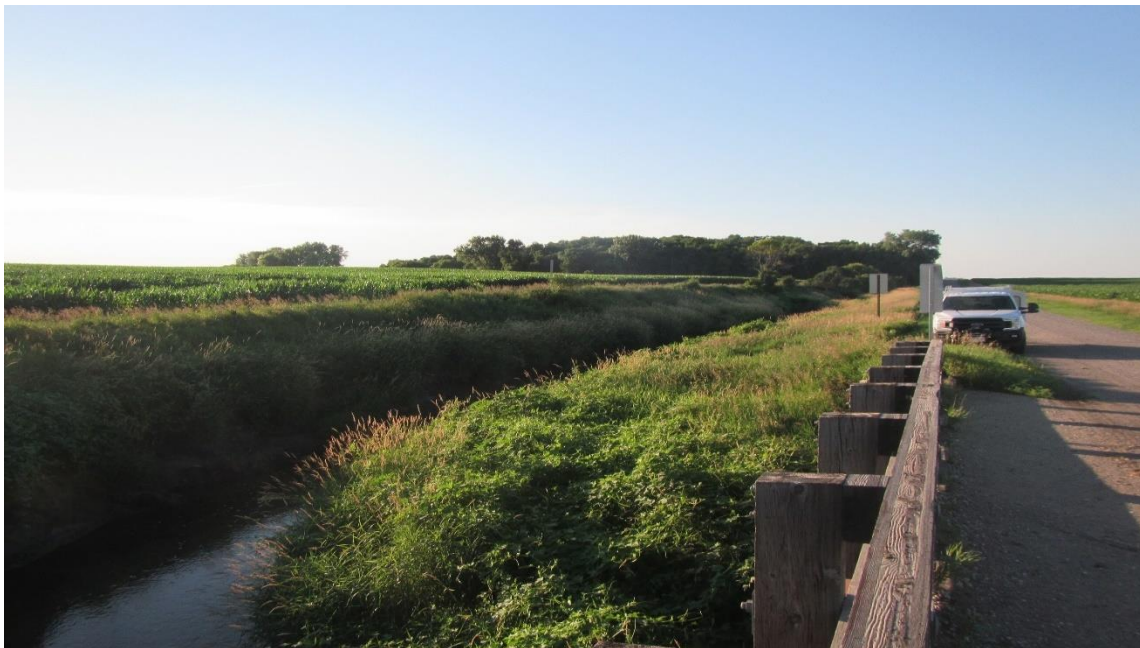
Figure 43. Photo taken near bio site 09MN039 showing channelized channel and drainage culverts.
