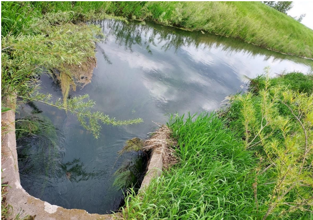
Figure 29. Culvert at the road crossing near bio site 09MN073.
