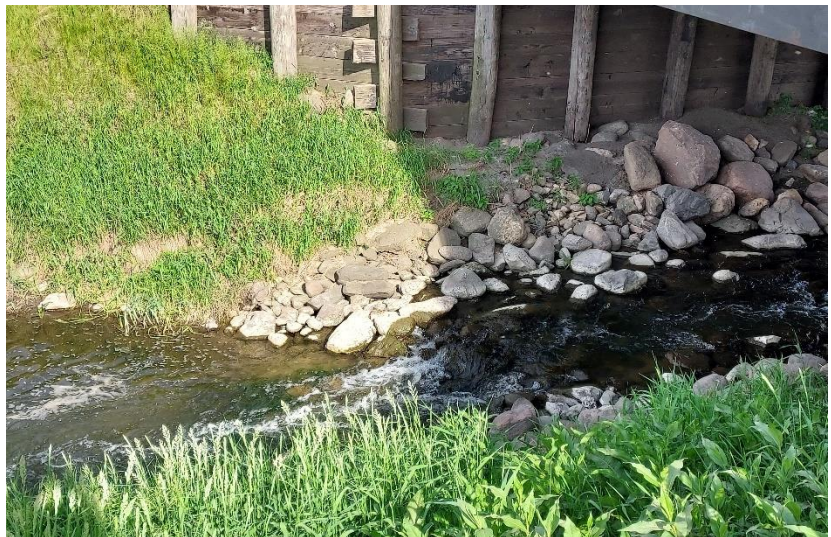
Figure 64. Photo of rocks placed under the bridge at road crossing near bio site 07MN049.
