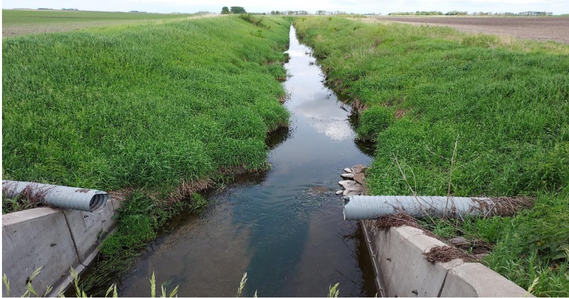
Figure 42. Photo taken from the bridge crossing near bio site 09MN040.
