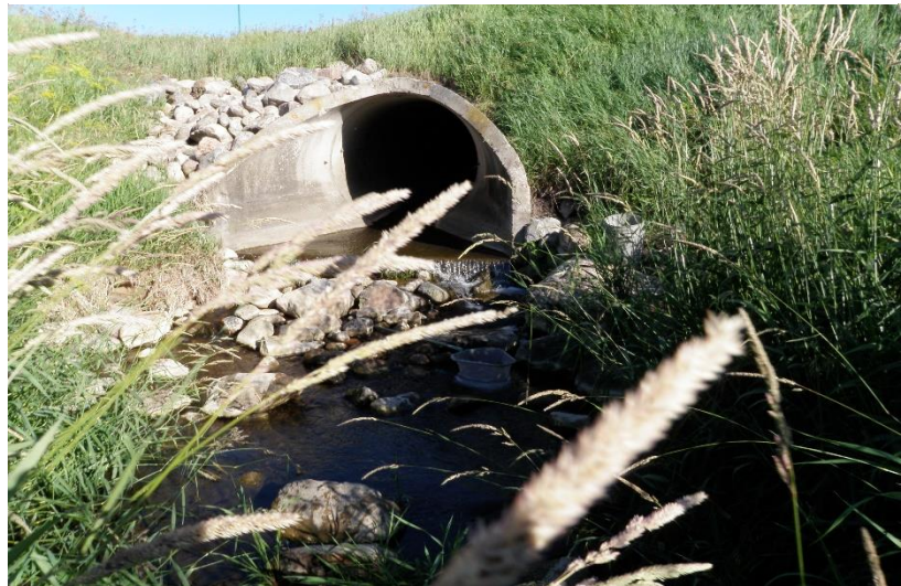
Figure 36. Photo of culvert underneath the road crossing near bio site 09MN048.
