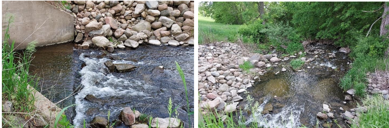
Figure 58. Photo of the culvert underneath the road crossing near bio site 09MN020 (left) and the artificial rock rapids just downstream of the culvert (right).
