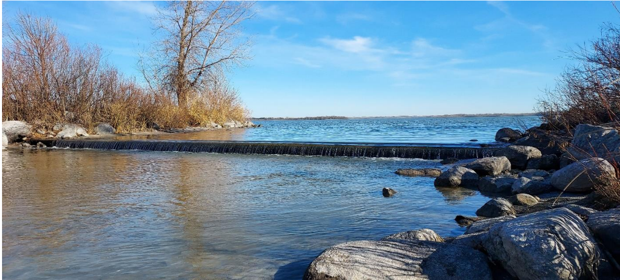
Figure 16. Lake water level control structure at the outlet of Lake Mary.
