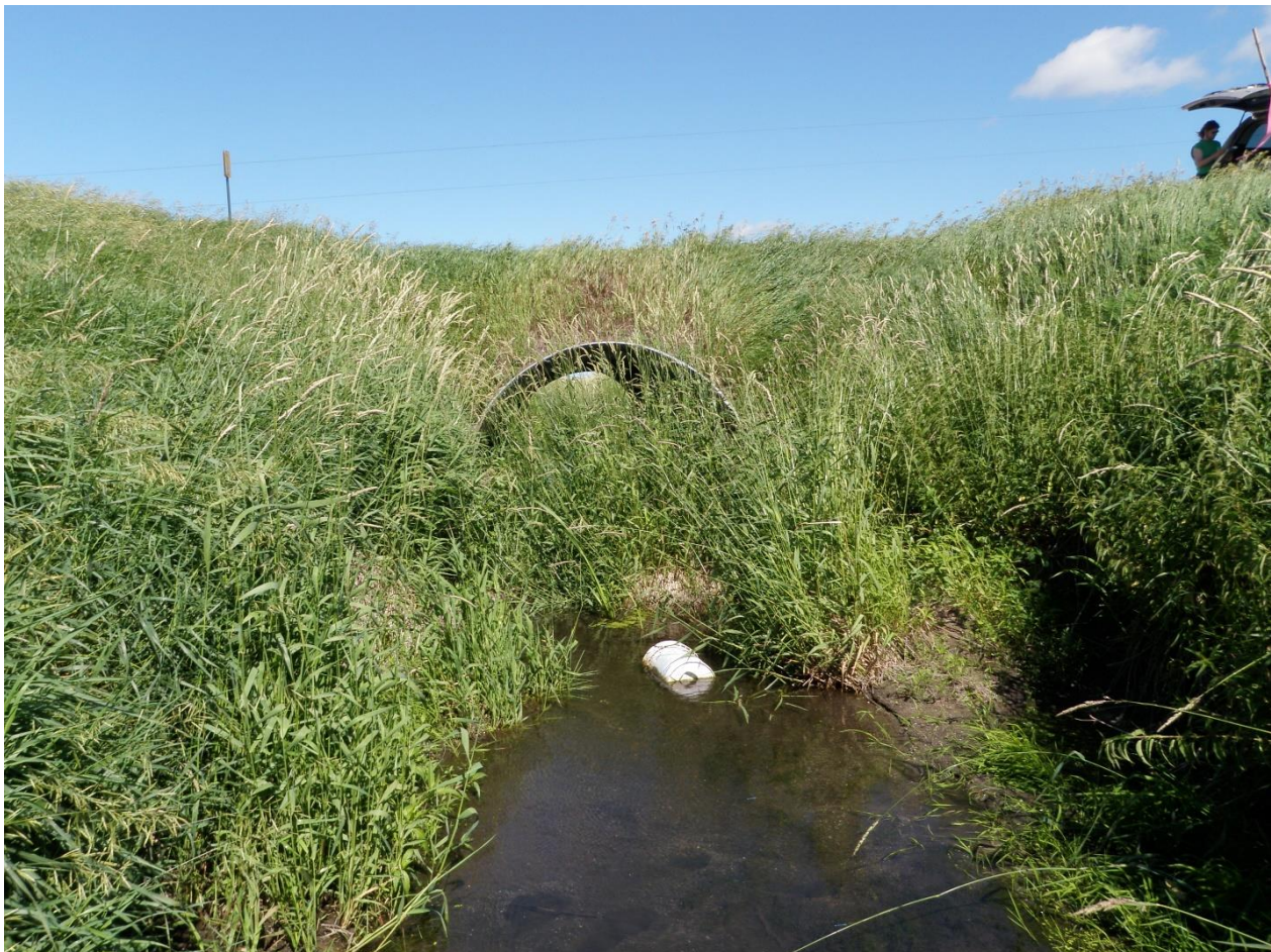
Figure 38. Culvert underneath road crossing near bio site 09MN046.
