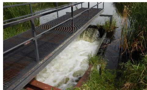
Figure 7. Dam on Pelican Creek (8/29/19)
