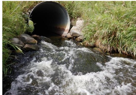
Figure 8. Velocity barrier from culvert
