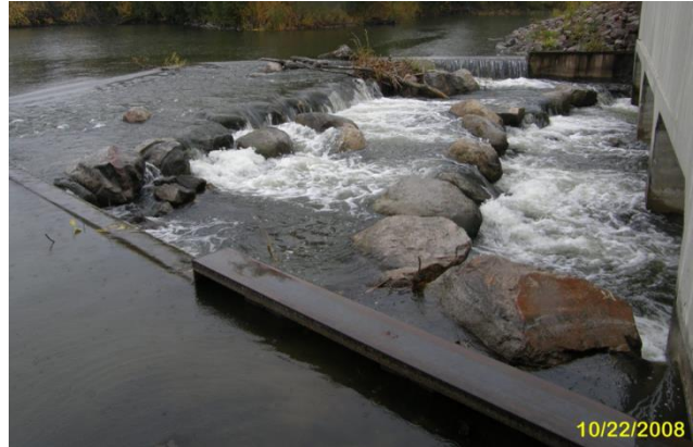
Figure 13. Barrett Lake dam (DNR).
