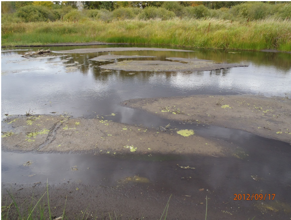
Photo 24. Sediment deposition at 10UM053 just above the Smokey Hills Road culvert
