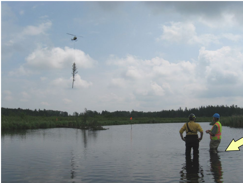
Photo 13. MDNR deemed that parts of the adjacent Straight River needed habitat enhancement due to the absence of structural habitat/cover and channel forming materials. Trees were imported and carefully placed to enhance the naturally bland, homogeneous channel morphology. MDNR Photo
