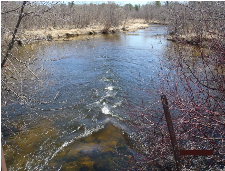
Photo 19. Old bridge structure at 580 th Ave., May 2013. High velocity occurs through the constriction between the concrete bridge abutments and a large scour pool results. A couple large suckers (~14") were seen on upstream side of bridge. Small species would have much difficulty passing through this level of water velocity.
