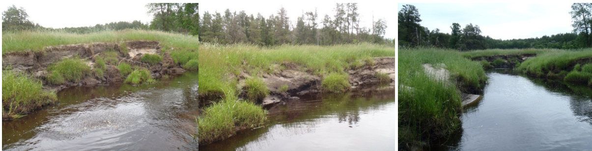
Figure 4.2.11: Photos of bank instability located downstream of Long Farm road near “2 nd Site” sampling location.
