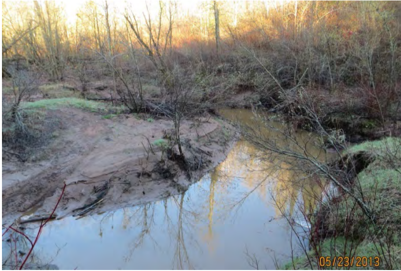
Figure 59. Eroding streambanks on Clear Creek
