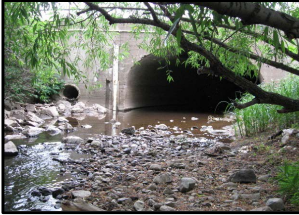
Figure 22c. Miller Creek outflows from an underground culvert that daylights at 26 th Avenue West in Duluth, MN. This culvert is not perched, but is representative of the habitat loss present in the urbanized setting.
