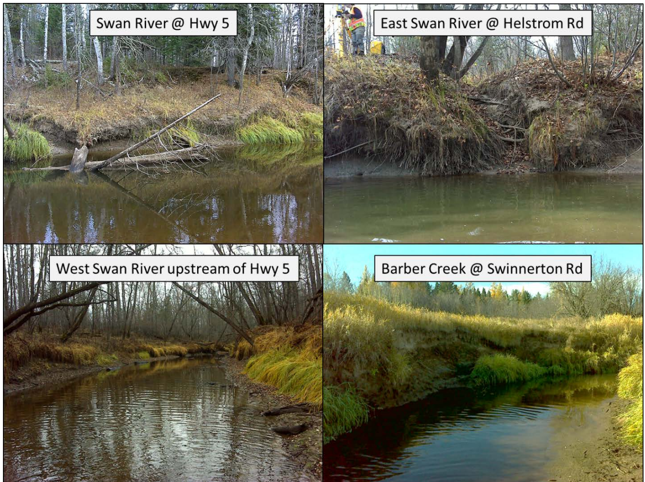
Figure 358: Examples of bank erosion and channel instability in the Swan River watershed
