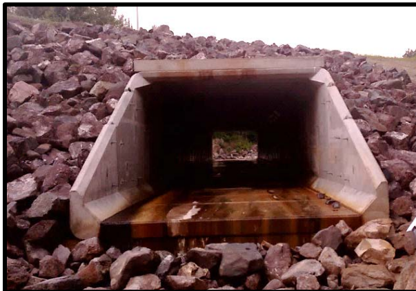
Figure 22a. Perched culvert on Kingsbury Creek at US Hwy 2 crossing, acting as a barrier to fish movement.
