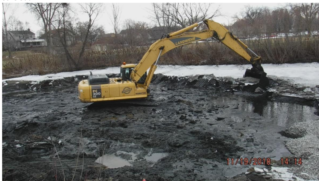
Figure 17. Dredging of the Stormwater Treatment Pond "Little George" – November 2018. Photo Credit – City of St. Cloud
