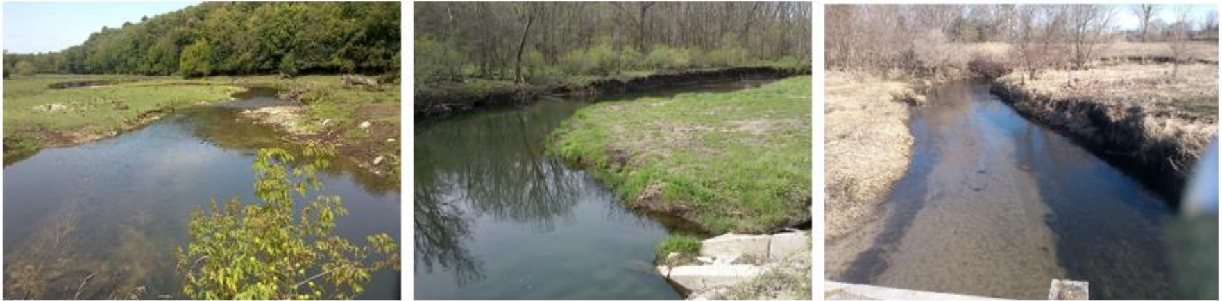
Figure A-5. Areas of severe bank erosion on Spring Valley Creek. From left to right: (S000-769/08LM006—looking upstream, S000-769/08LM006—looking downstream and upstream of S000-772 at trail/bridge crossing).
