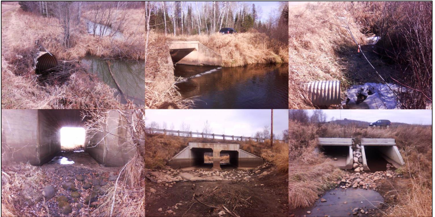
Figure 25: Examples of connectivity barriers. Pictured are a 4' high beaver dam built at a crossing (top left), slightly perched culvert with a very shallow low flow water depth (top center), >1 foot perched culvert (top right), and low flow disappearing in cobbles (bottom three photos)
