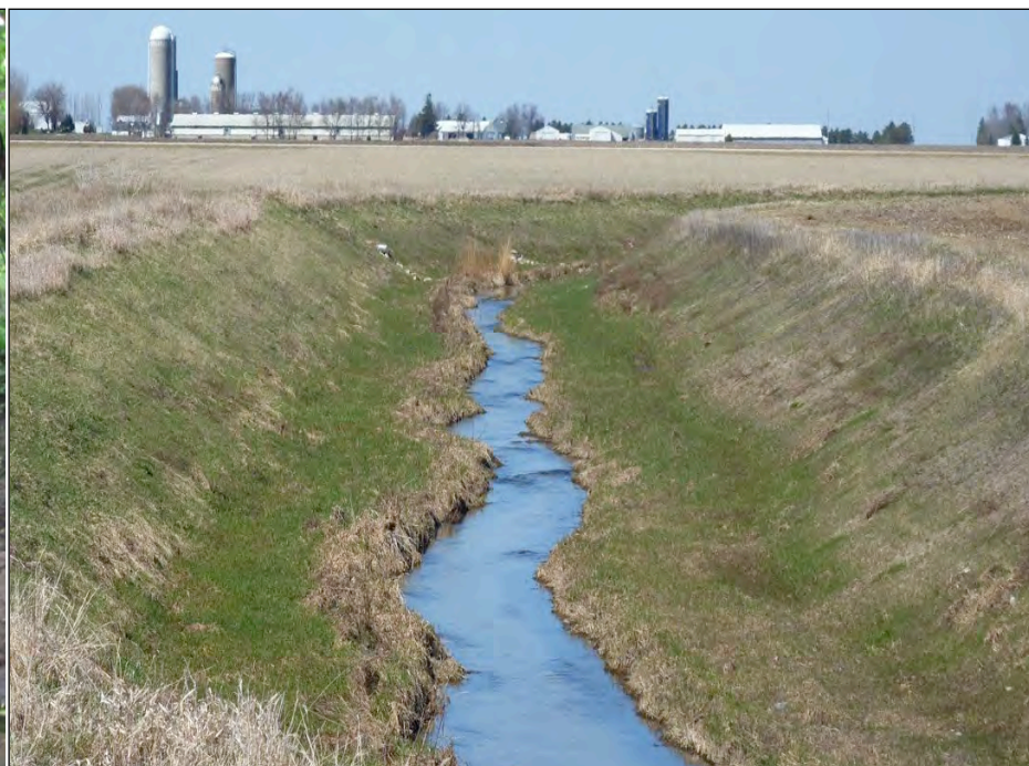
Image2: Mullenbach two-stage ditch after construction in Spring 2010
