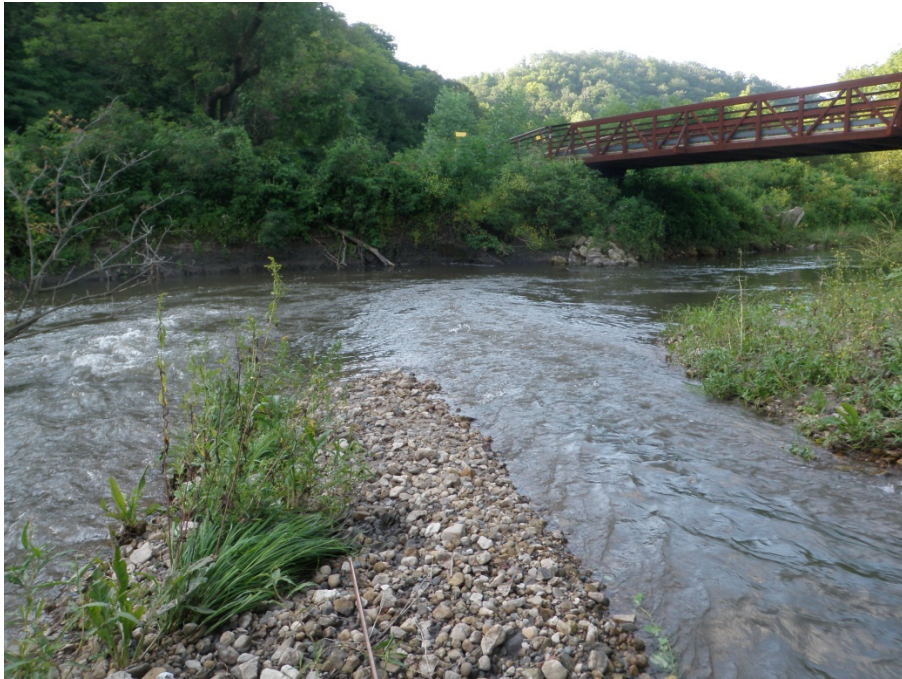
Image 18: Lateral riffle deflecting flow into the outer bank by new ATV bridge on Belle Creek. Image taken on August 4, 2011 before large storm event and high flows caused more severe bank erosion in fall 2011 and 2012.
