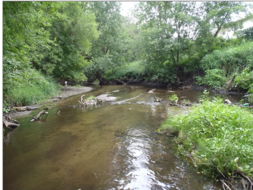
Image 5: Station 10UM032 on Shingle Creek. Stream is overwidened with severe bank erosion and excess sedimentation infilling habitats.
