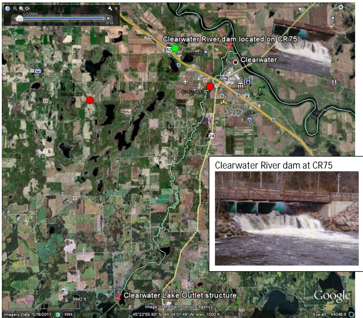
Figure 81: Clearwater River reach below Clearwater Lake outlet and the Mississippi River. This reach has a dam located at CR75 which prohibits fish passage and controls channel hydraulics
