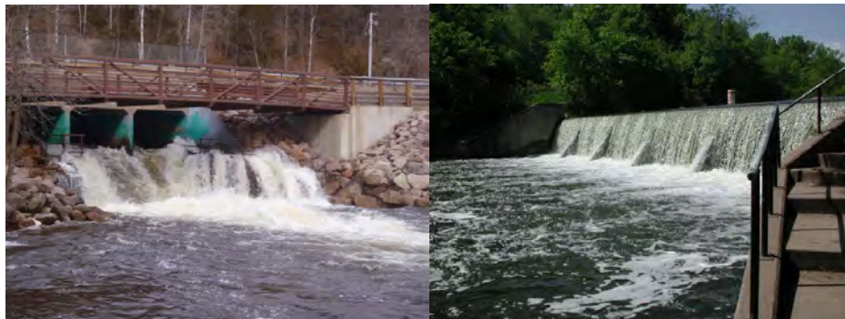
Dam at CR75 nr City of Clearwater
