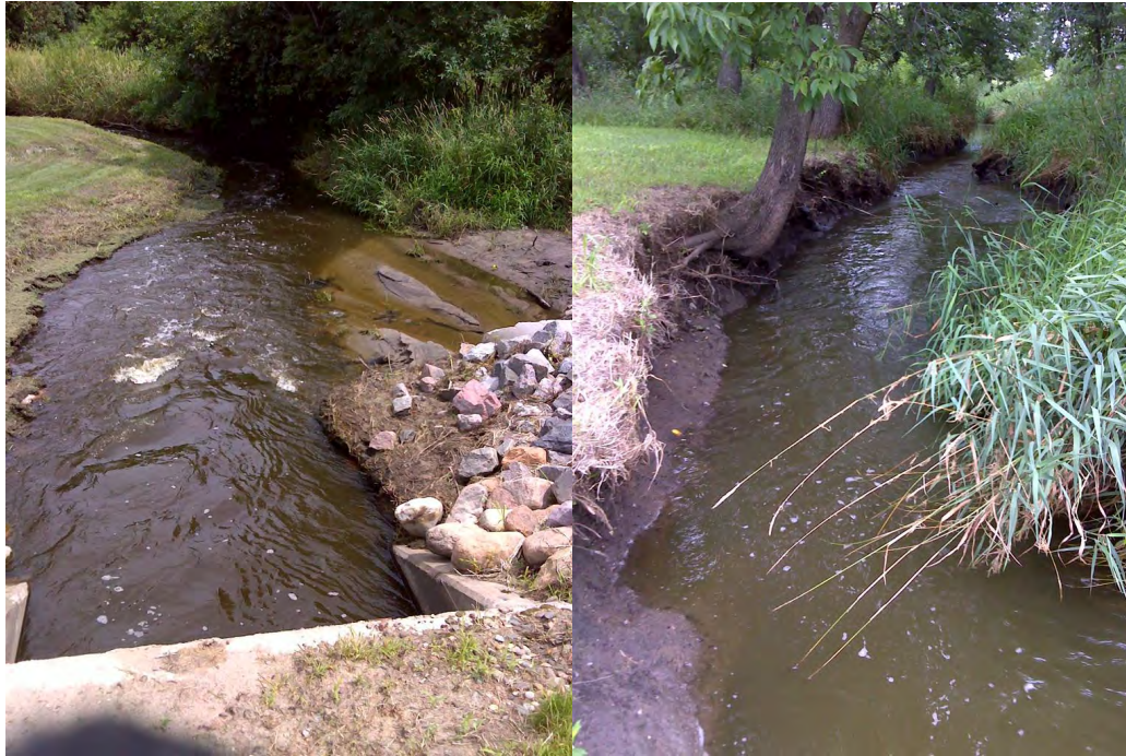
Figure 98: View of downstream stream section below the Nabor Avenue culvert. This site has a double culvert, one box and one arch culvert. The arch culvert is filled with sand and only carries flow during high flow events.
