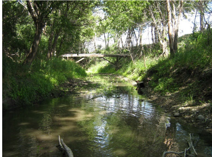
Monitoring station 07UM099 (07010204-563)
