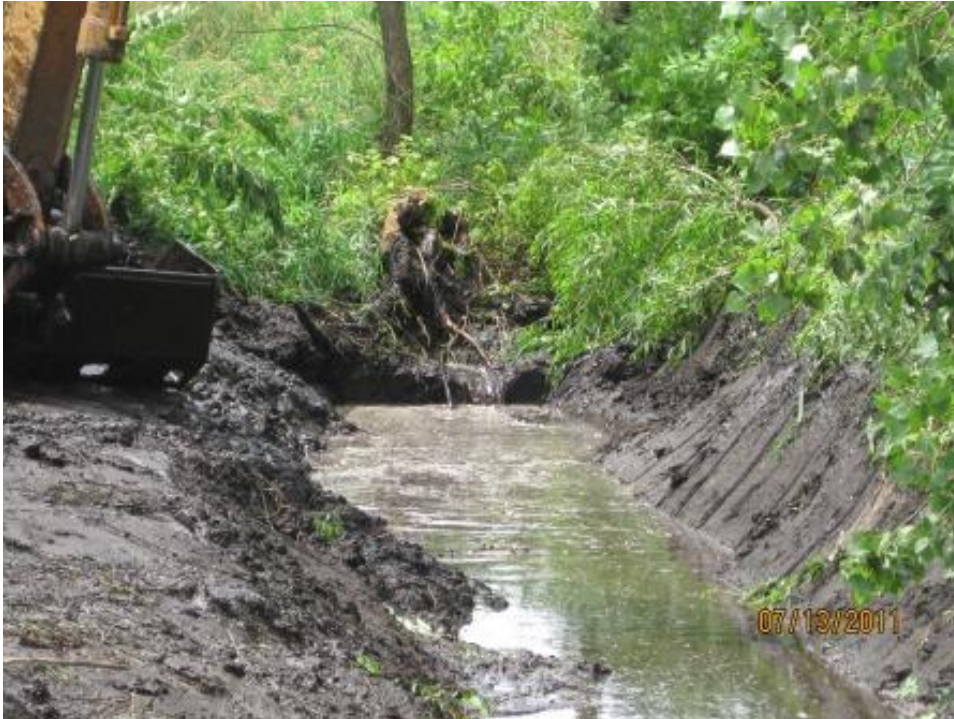
Figure 37. Channel in the process of being dredged.
