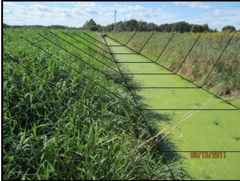
Figure 52. Geometry of constructed agricultural ditches across CCWD.
