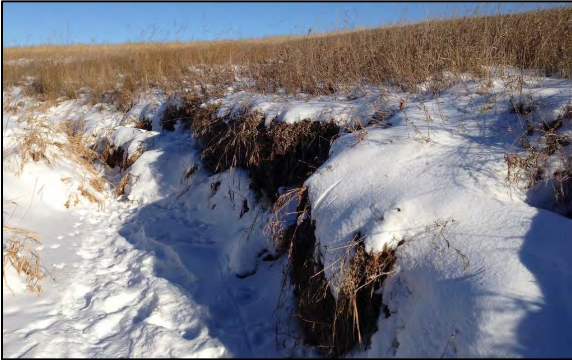
Figure D-6. Sunset Bay tributary streambank erosion location SB2R.
