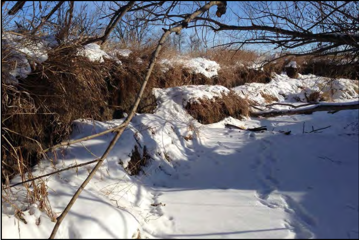
Figure D-3. Okabena Creek streambank erosion location OKA13.
