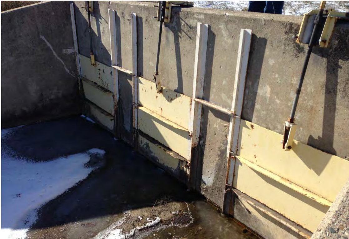
Figure 2-3. Okabena Creek bypass flood gates at Oxford Street.
