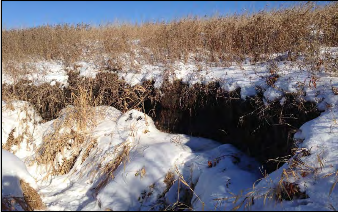
Figure D-5. Sunset Bay tributary streambank erosion location SB1R.
