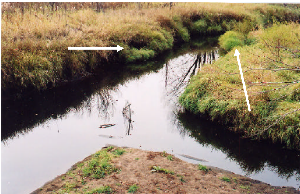
Figure A4. Downstream of site 3. A sandbar associated with excessive sediments and bridge pylons (MN23). Actively eroding banks insufficiently supported by reed canary grass are highlighted with white arrows.
