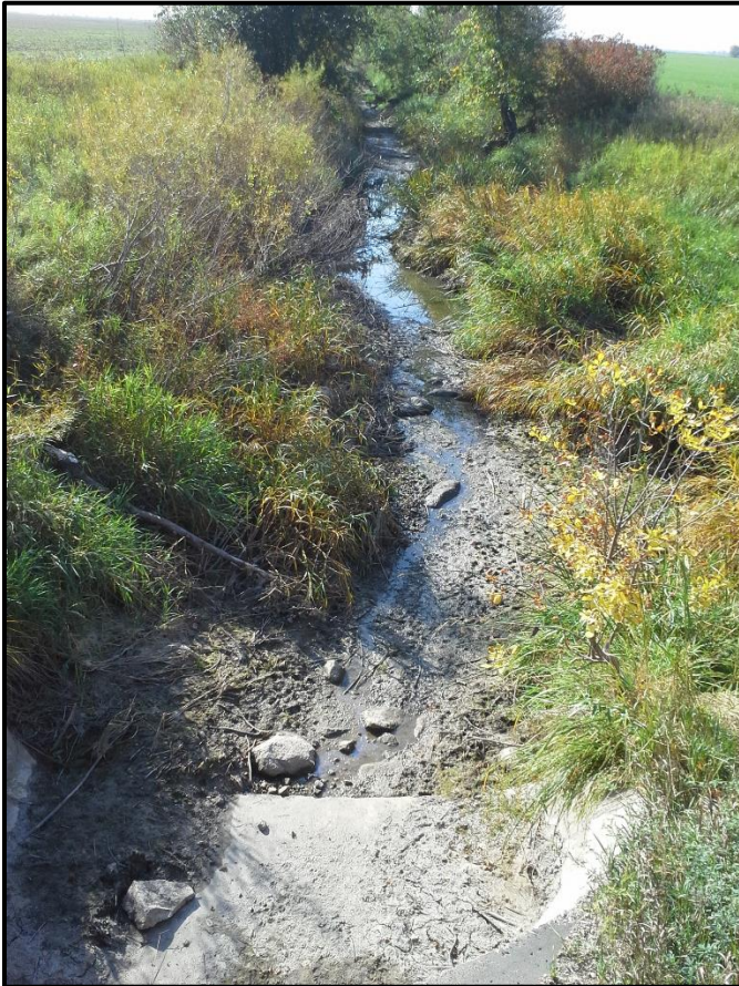
Figure 4-63. No-flow conditions in the Black River at 120th St. NW (S003-948).
