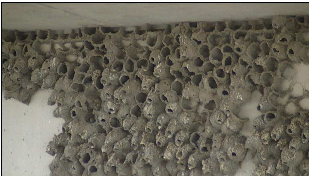
Figure 4-16. Cliff swallow nests under a bridge.
