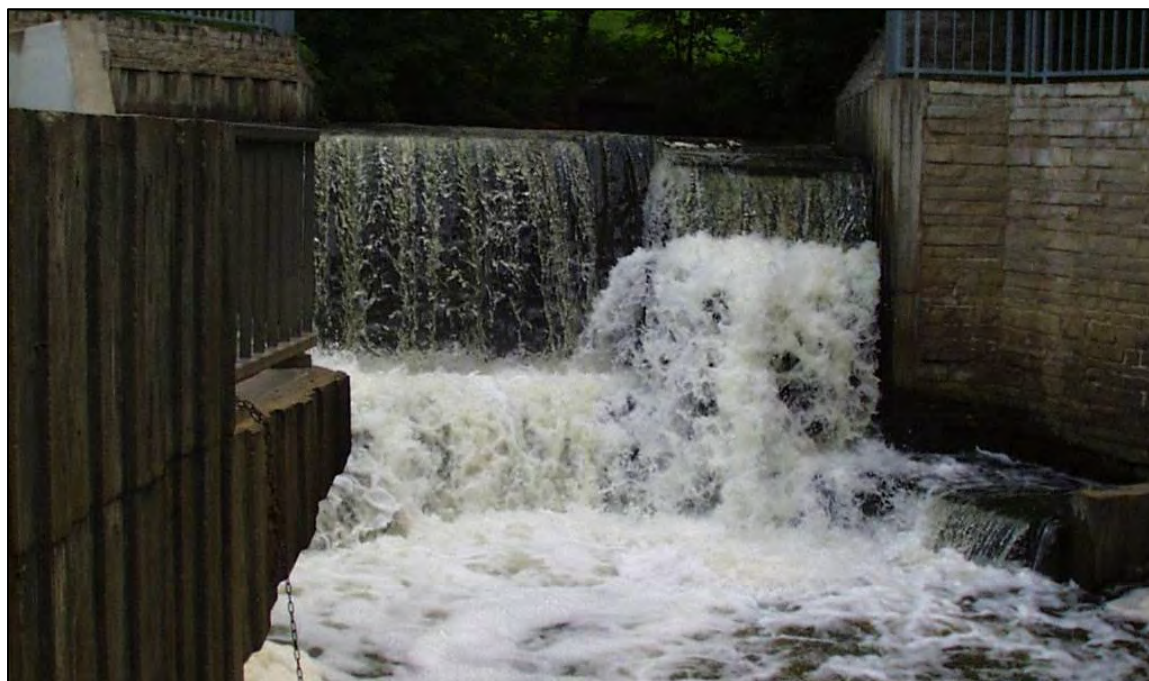
Figure 3.16. Drop structure in Webber Park that disconnects Shingle Creek from the Mississippi River.
