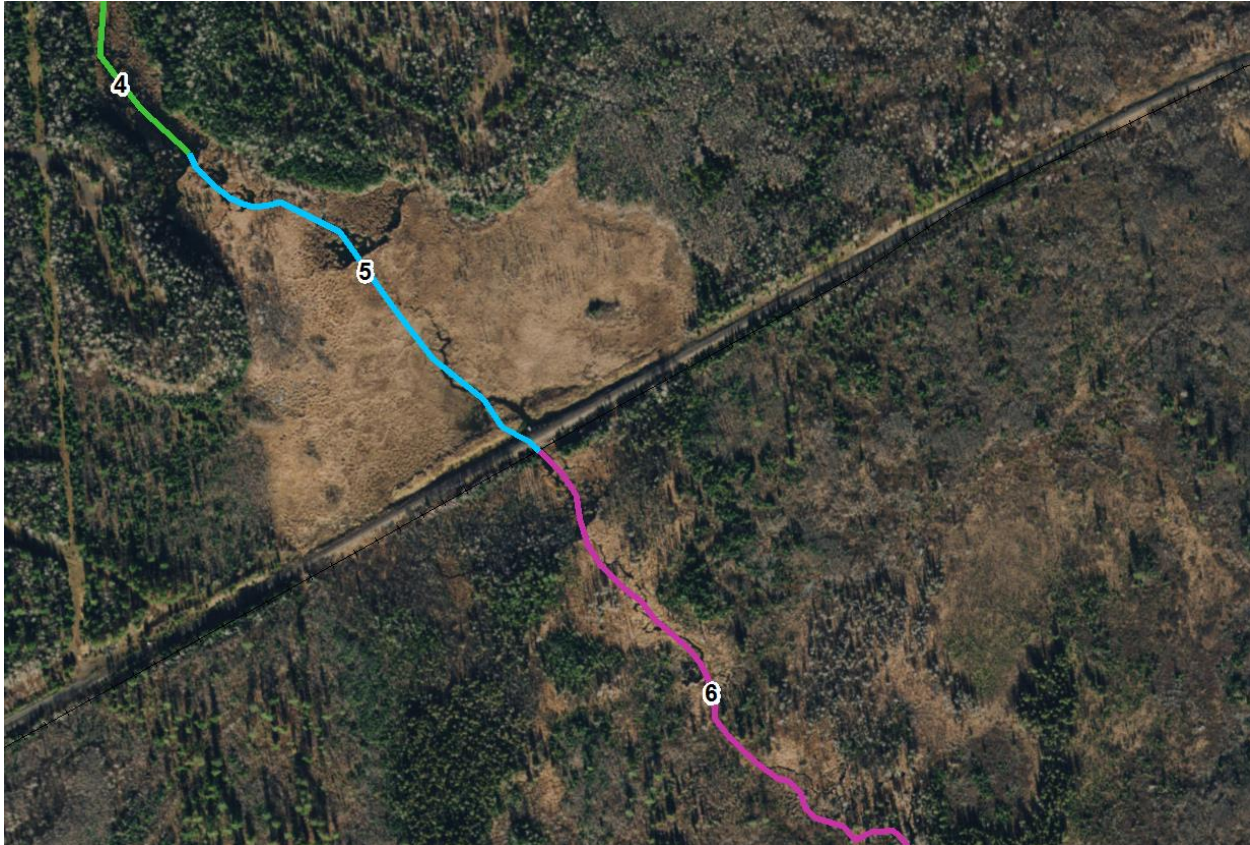
Figure 27. Aerial imagery of Reach 5 and the impact of ponding upstream of the perched culvert.
