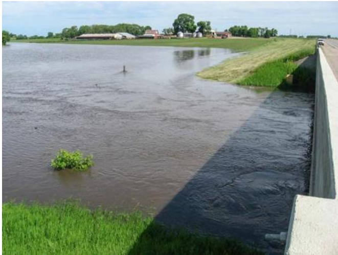
Figure 8. Hawk Creek flooding along Hwy 23 bridge between Maynard and Granite Falls in June 2014
