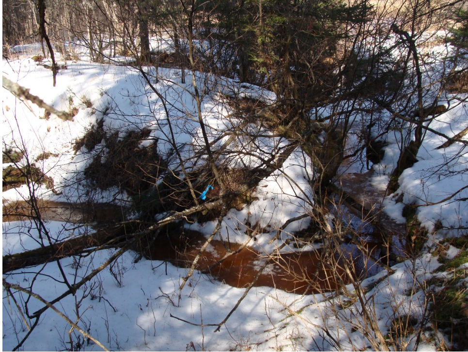
Figure 5. A steeper portion of ravine located on the downstream end. Note that the downstream locations are typically forested rather than open, reducing the probable erosion rates. The highest erosion rates were predicted for the steeper, downstream ends.
