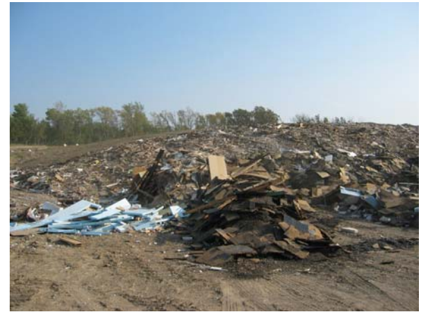
Demolition Cell at the Fergus Falls Landfill. Photo by Kathy Holland-Hanson
