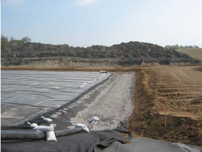
Liner construction at NE Otter Tail Landfill. Photo by Kathy Holland-Hanson
