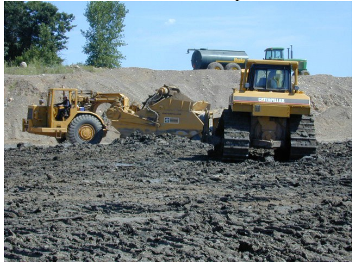
Liner construction at the Morrison County Landfill. Photo by Kathy Holland-Hanson
