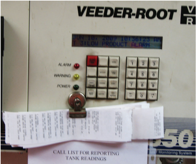
Photo 1: Examples of Automatic Tank Gauges (ATGs)
