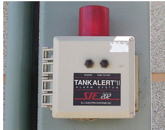
Photo 11: Examples of overfill alarms. Some alarms only come with horns (left) and some also feature warning lights (right).
