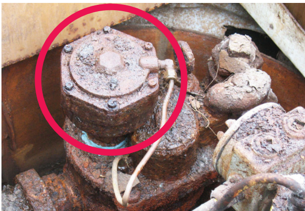
Photo 4: Examples of mechanical line leak detectors (MLLDs).
