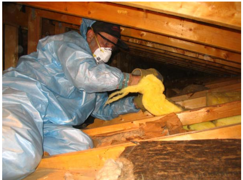
Adding batt insulation in the attic reduces heat loss and increases energy efficiency. Photo from the Minnesota Department of Commerce
