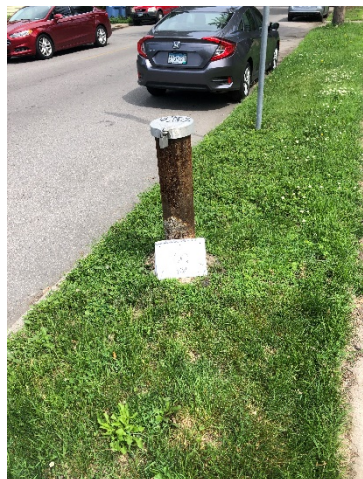
Photo 23- Well QQ. ~1 1/2" well casing, plug present, no bollards.
