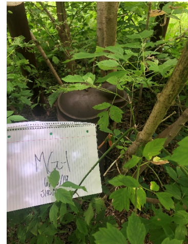
Photo 16-Well MG-1. Hidden under vegetation and behind a tree. Two bollards present, one appears to have been backed into and is slightly bent.
