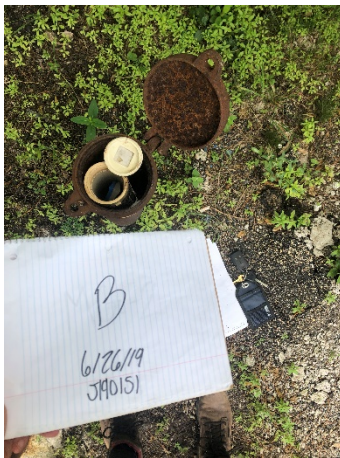
Photo 15- Well B. - ~2" PVC well casing, plug/cap present, two bollards and surrounded by fence to the south
