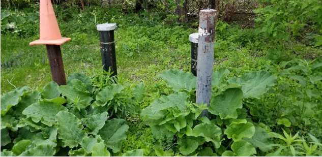
Photo 13- Well 311 GD and 311 GS. No damage noted.
