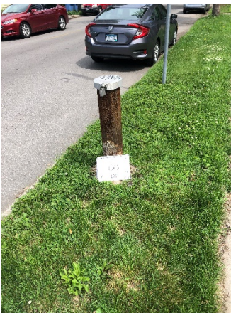
Photo 5 Well QQ. 1 1/2" well casing, plug present, no bollards.
