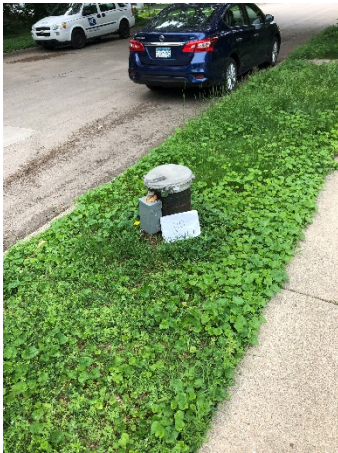
Photo 3 Well 110. No damage noted.
