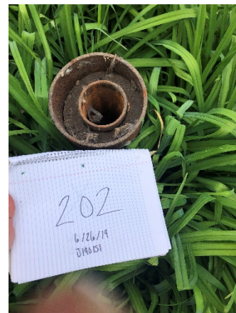
Photo 6 Well 202. 4" steel well casing, surrounded by vegetation,
