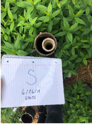
Photo 25- Photo 24- ~2" PVC well casing, plug/cap present, three bollards. No apparent damage.
