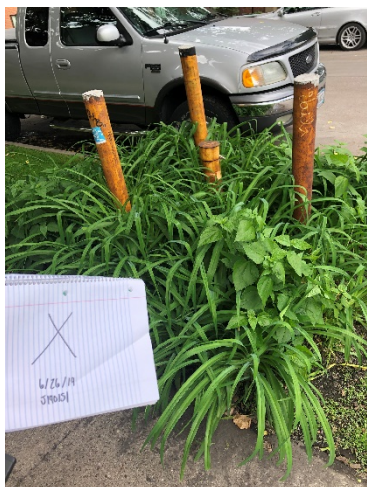
Photo 35- Three bollards, unable to remove lock.
