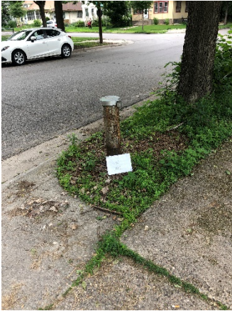
Photo 1 Well W located at 22 nd and Talmadge. PVC well casing present. No bollards.
