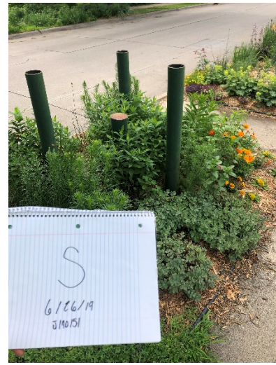
Photo 26- Photo 24- ~2" PVC well casing, plug/cap present, three bollards. No apparent damage.
