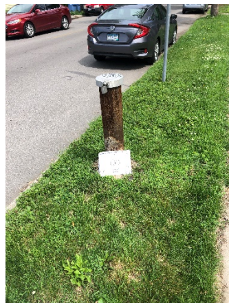
Photo 4 Well QQ. 1 1/2" well casing, plug present, no bollards.
