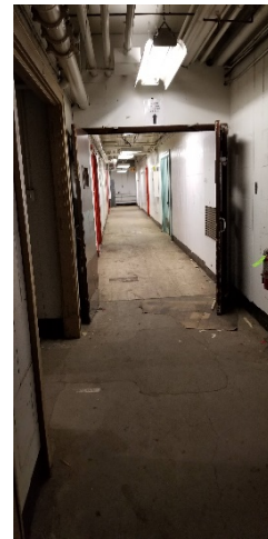
Photo 4. Tunnels of Building 10.
