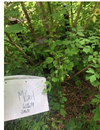
Photo 18- Well MG-1. Hidden under vegetation and behind a tree. Two bollards present, one appears to have been backed into and is slightly bent.
