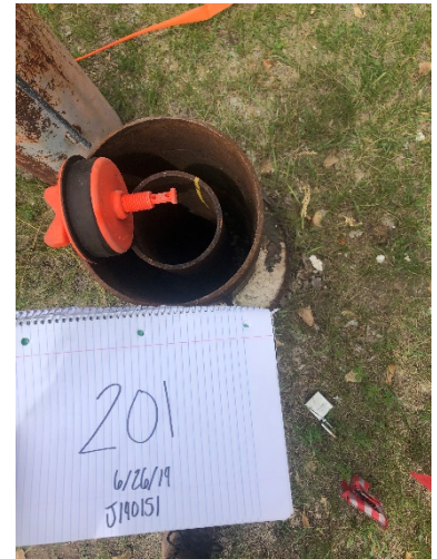
Photo 10 Well 201. 4" steel well casing, plug present, no bollards. Area under construction at time of inspection. No damage noted.
